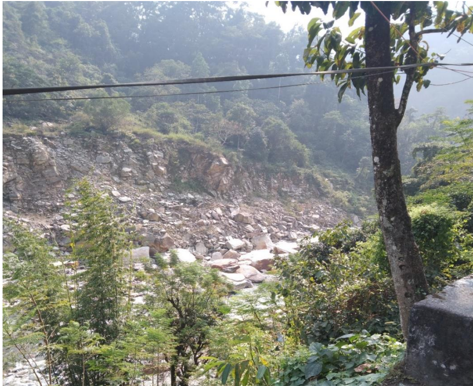
Figure 2.5. Bank failure in the Rangit at Legship area (27.279 N 88.277 E)
