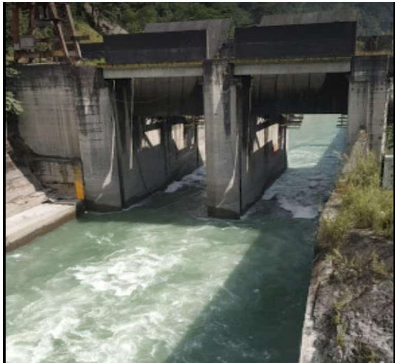
Figure 2.12. Teesta IV dam upstream of Singtam causing diversion of river channel.
