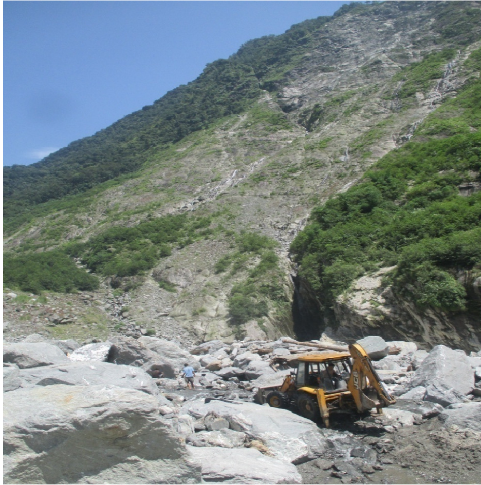
Figure 5. 5 Upper Dzongu Mantam Landslide maintenance work
