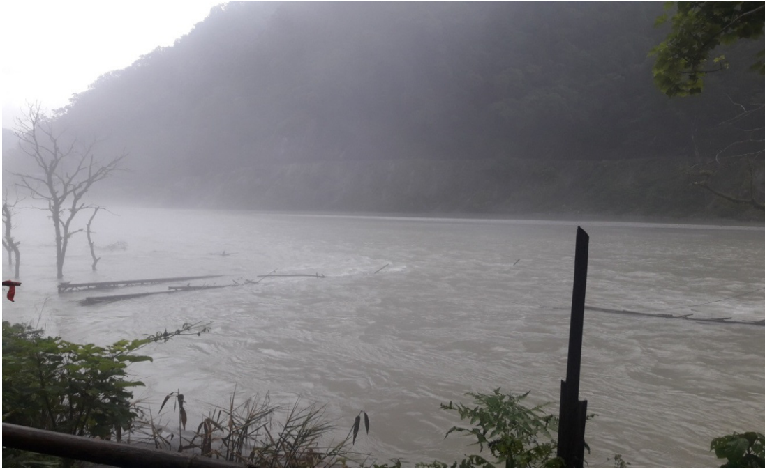
Figure 5.4. Mantam Bridge Collapsed during Rainy Season
