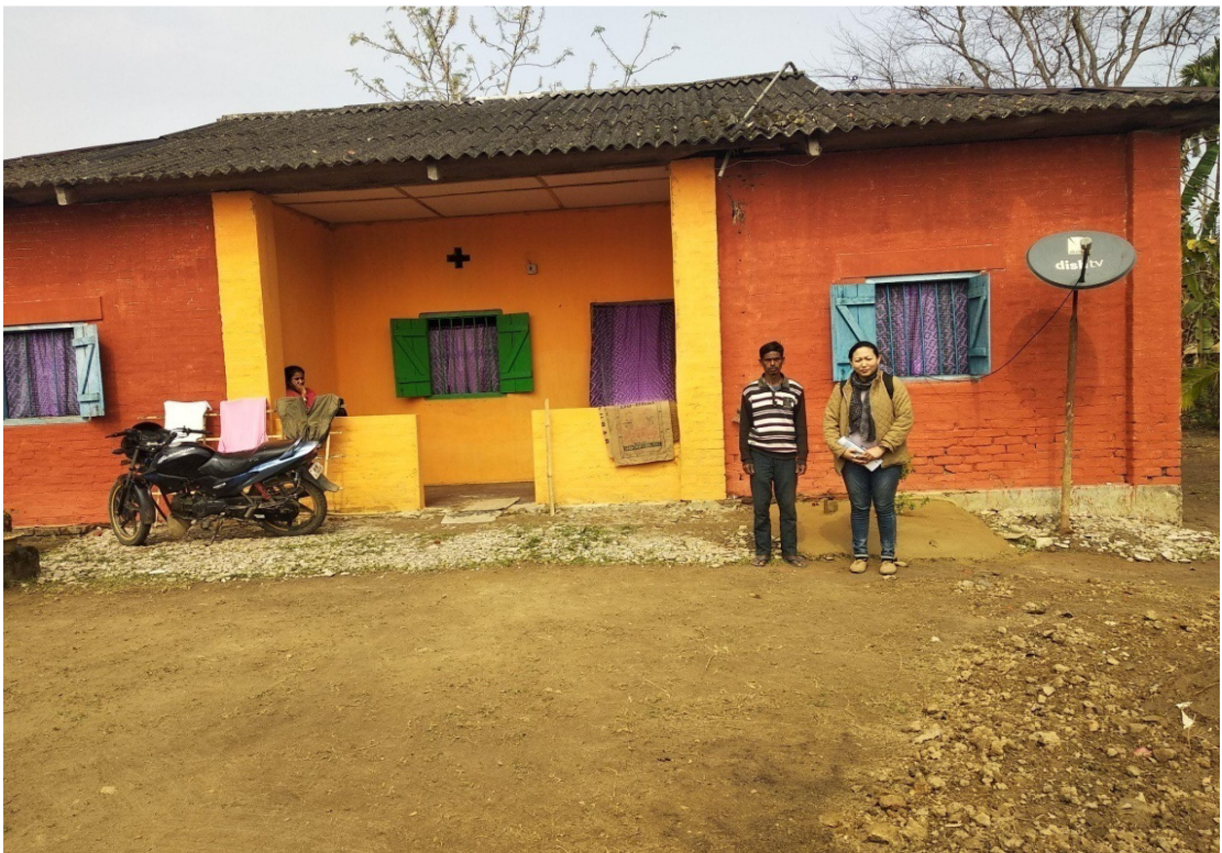
Picture: Pakka house provided to the tea garden worker by the Nalini Tea Garden. (Field Survey)
