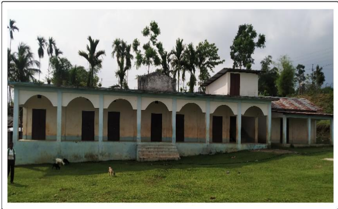
Fig.3.1: Primary School of Carri Line, picture taken on 22.04.2022.
