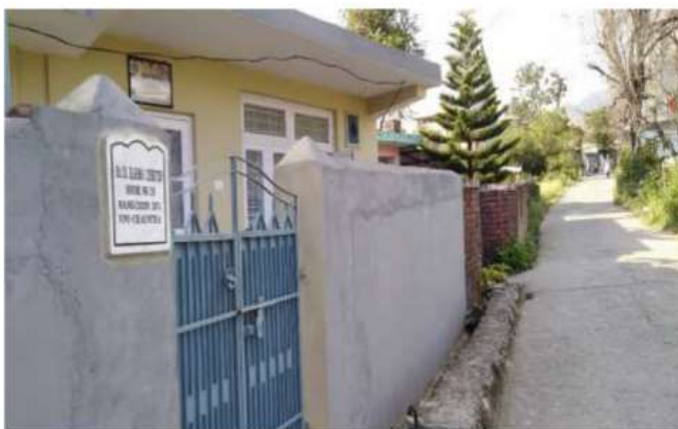
Figure 5.7: Pakka houses of Tibetan settlement of Bir Chauntra Tibetan Settlement (Nangchen) (Photo taken by the scholar on date 04.10.2018)
