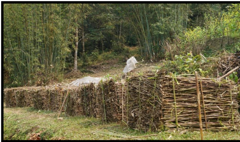
Plate No.33: Above ground perforated pits (1 m 3 dimensions) using bamboo
