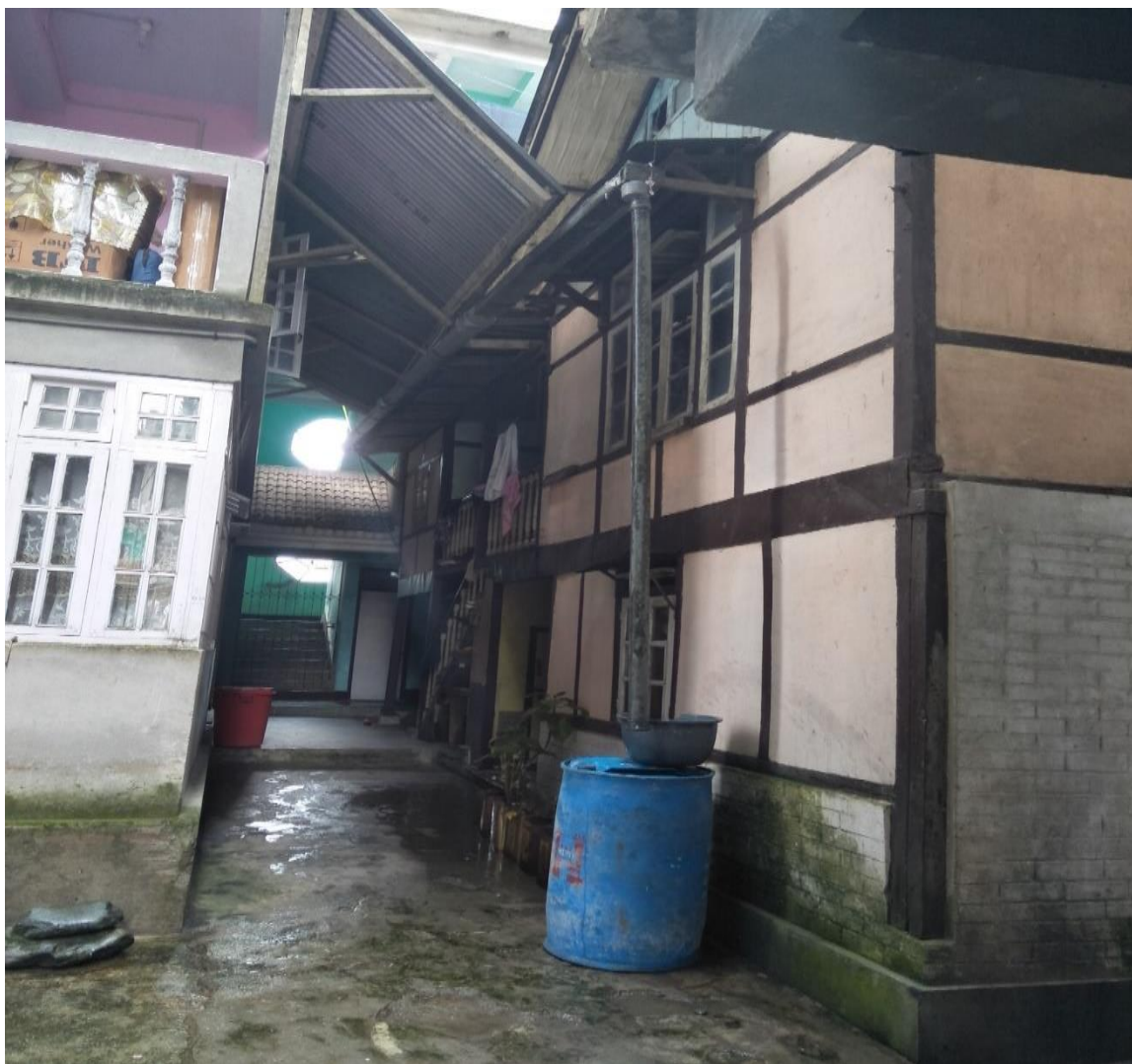
Figure 6.1 The household practicing roof water harvesting in urban East Sikkim district
