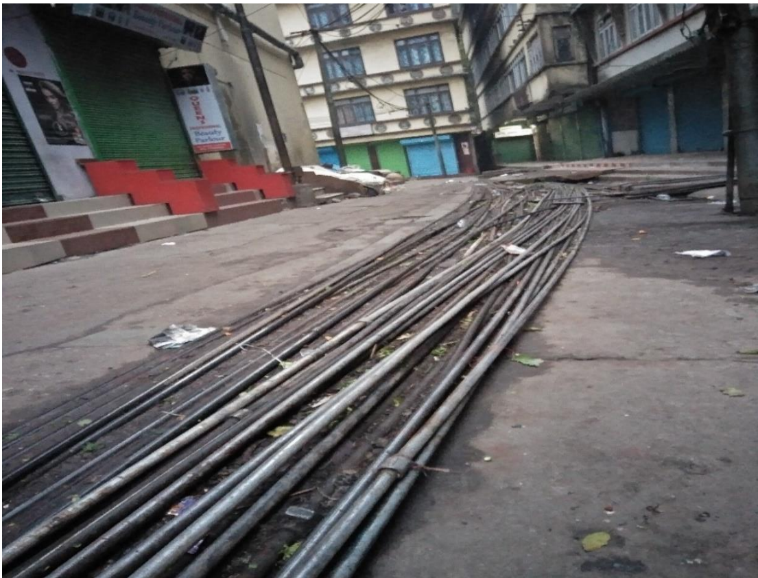
Figure 5.3: Household Water Connection through Pipelines Provided by the PHE Department
