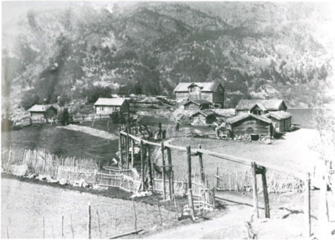
Fig. 12 Half-open wooden pipe to lead irrigation water at Søre Neset farm, Vågå, E-Norway ( Photograph Hans Joramo/De Sandvigske Samlinger Maihaugen); released under a Creative Commons Attribution-NonCommercial-NoDerivatives 4.0 International License
