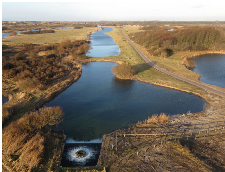
Fig. 12 Infiltration point of surface water from the lake IJsselmeer into the infiltration channels in coastal dunes area of Castricum. Photograph: T. Kisjes
