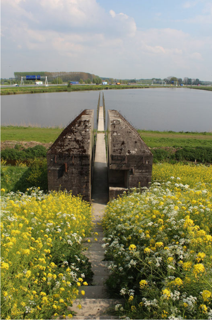
Fig. 6 Cut-through bunker 599 as part of the water storage and preservation of a bunker landscape. Courtesy Verschuure-Stuip 2014; released under a Creative Commons Attribution-NonCommercial-NoDerivatives 4.0 International License
