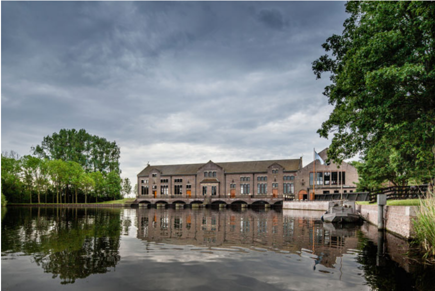
Fig. 7 View of the World Heritage listed steam pumping station (Woudagemaal) in the city of Lemmer, the Netherlands. Image courtesy of Daniel Hartog; all rights reserved
