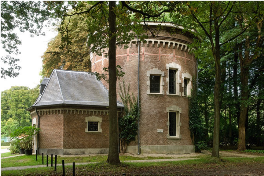
The oldest watertoren of the Netherlands (constructed 1678–1683), served the fountains of the gardens of Paleis Soestdijk, a former palace and hunting lodge of the Dutch Royal Family. The water reservoir was supplied by means of a windmill and a horse drawn mill. Source Beeldbank Rijksdienst voor het Cultureel Erfgoed; released under CC BY-SA 4.0 Photographer Jan van Galen
