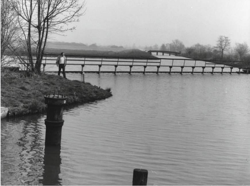
Fig. 14 Drinking water canal ( Waterleidingkanaal ) transporting seep water from Bethunepolder to the Loenderveenseplas for natural purification (ca. 1988). Source Het Utrechts Archief; released under a Creative Commons Attribution-NonCommercial-NoDerivatives 4.0 International License
