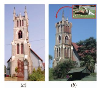
Figure 14. Collapse of brick spires of Mac Farlene Church at Kalimpong (MSK-V): (a) before the earthquake (Photo: http://mntravelog.com/tag/macfarlane-memorial-church/) and (b) after the earthquake.
