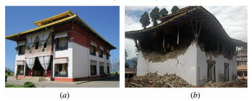
Figure 13. (a) Satisfactory performance of King's monastery in Gangtok (*MSK-VI*) and (b) partial collapse of Ringhem Choling Monastery at Mangan (*MSK-VI*).
