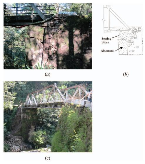
Figure 6. (a) Failure of seating block overhanging the abutment of Plaekhola Bridge, (b) schematic of the failure of seating block at Plaekhola Bridge and (c) damage to the wing wall of steel truss bridge on Raykhola.
