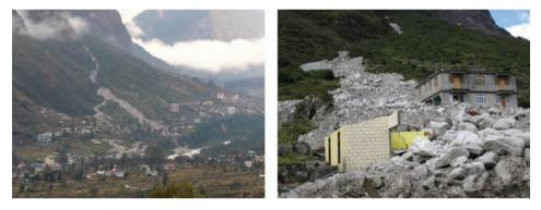
Figure 3. Damage caused due to rockslide and mudslide at Lachung (MSK-VIII).
