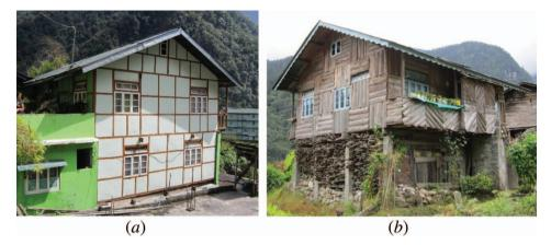
Figure 7. Traditional construction type: (a) Ikra house and (b) Shee-Khim house.
