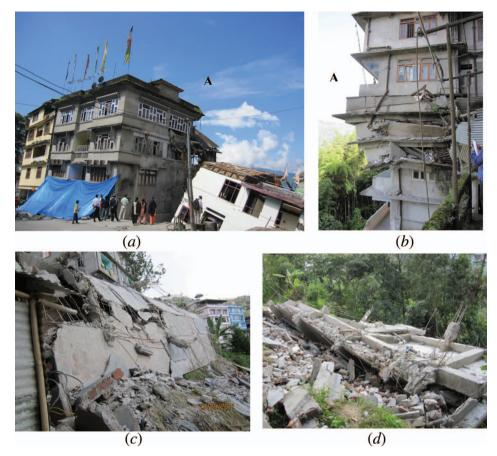
Figure 5. (a) Collapse of two multi-storey buildings at Balwakhani in Gangtok (MSK-VI); (b) view of building A, in figure 5a, from backside; (c) and (d) collapse of a five-storey building at Lumshey Basty in Gangtok.
