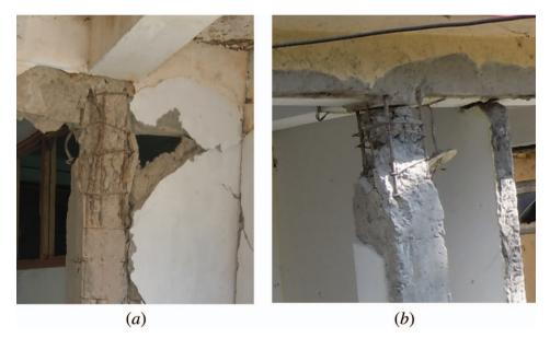
Figure 8. (a) and (b) Typical failure at column ends (widely spaced stirrups with  $90^{\circ}$  hooks, cold junction at the column top, poor concrete quality).
