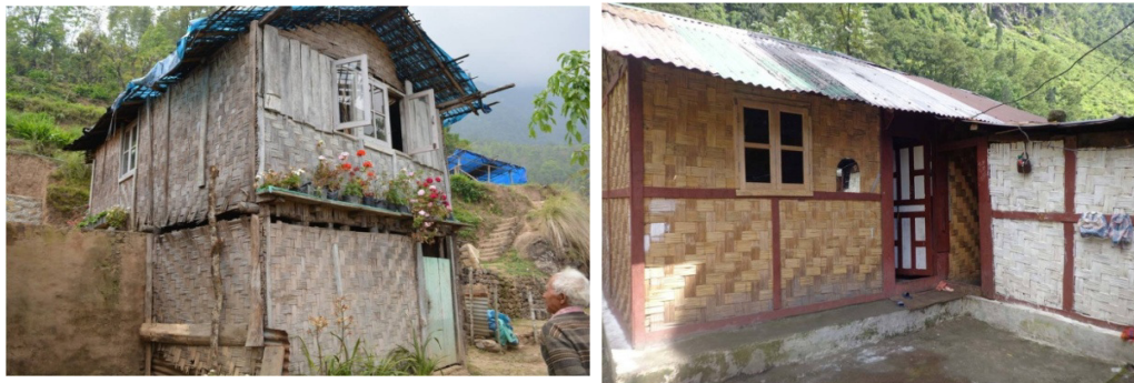
Plate IV.9: Chitra house in Sombarea (West Sikkim) and Chungthang (North Sikkim)
