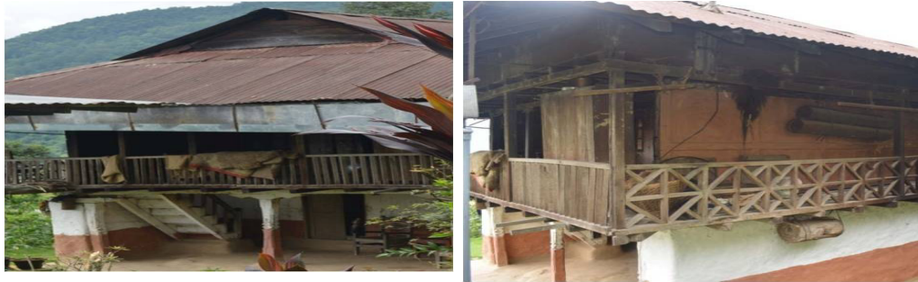
Plate IV.6: Over 50 years old Chaukat house in Assembleney, East Sikkim
