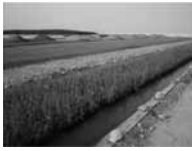
Shell: Produced Water Treatment Using Reed Beds, Nimr, Oman
