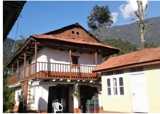
Image 2.7.Typical house in Daramdin
