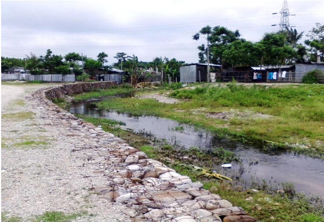
Rural connectivity between a village and the main road, constructed by MGNREGS beneficiaries in Gossainpur Gram Panchayat
