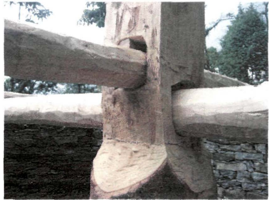
Carved poles for traditional house under construction
