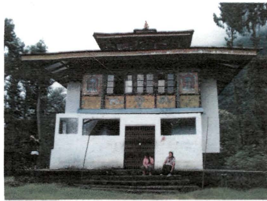
Locked Tingvong monastery
