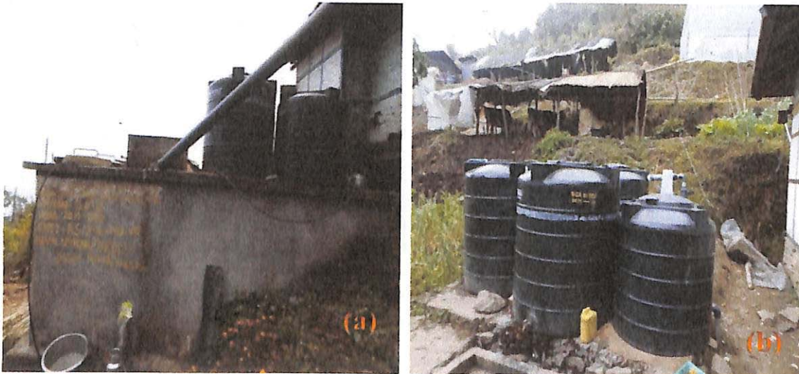
Plate IV.3: A roof-water harvesting in Budang village.
